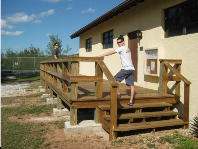
New Deck on Maintenance Building.
